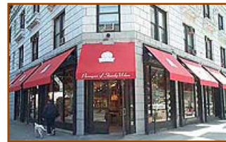
A good example of mounted awnings placed below the horizontal expression line.
