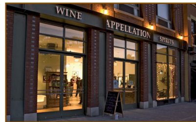
An example of large windows providing significant visibility into the building.
