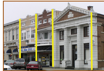
Desired vertically-proportioned buildings.
