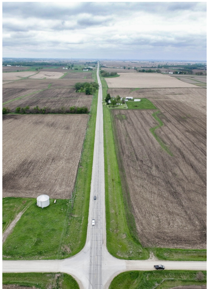
Highway 38 & 330th St. Intersection Looking North
