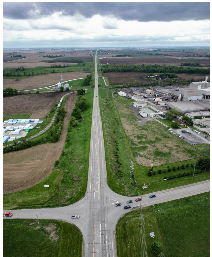
Intersection at Highway 38 & W 3rd St. Looking South
